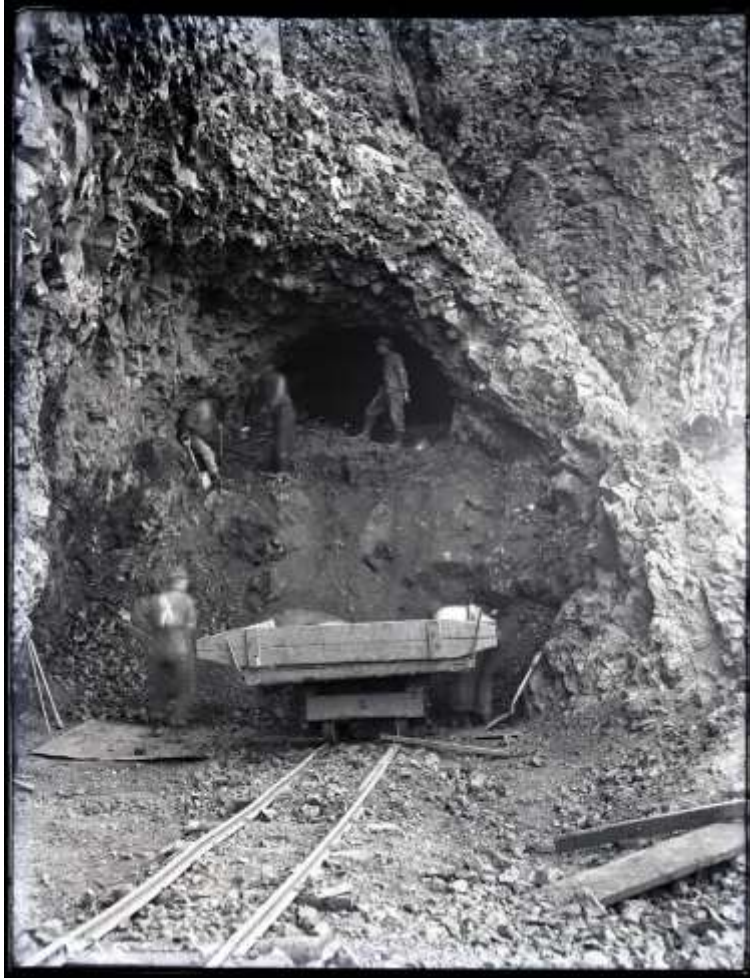
Albert H. Barnes (American, 1876–1920), Tunnel Construction , c. 1914; Gift of Samuel Hill, Collection of Maryhill Museum of Art, 1938.1.236
