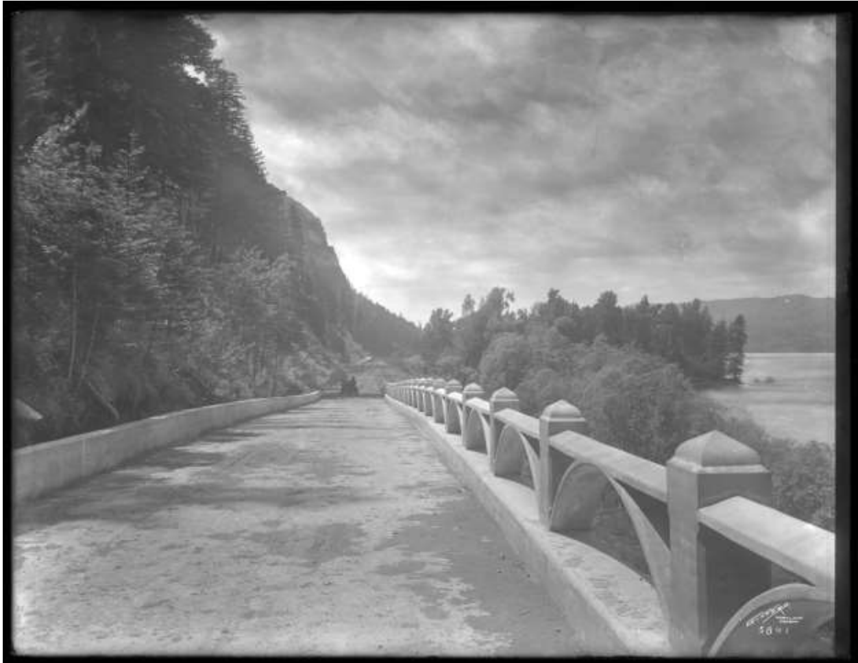
Benjamin A. Gifford (American, 1859–1936), East Multnomah Falls Viaduct, Columbia River Highway , c. 1915; Photo File 271-G, Neg. No. Gi 5841, Oregon Historical Society Research Library, Portland
