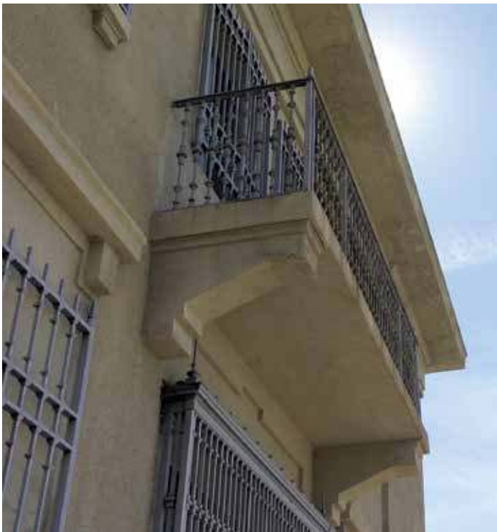
The original historic museum building has elegant in the simple understated architectural details that include balustrades, cornices, balconies and grill work. Photo by Scott Thompson.
