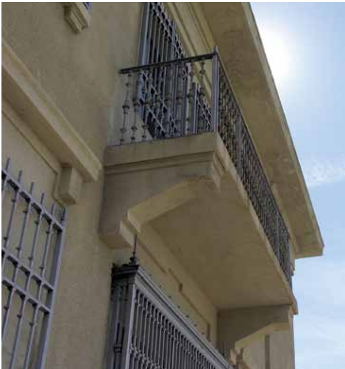
The original historic museum building has elegant in the simple understated architectural details that include balustrades, cornices, balconies and grill work. Photo by Scott Thompson.
