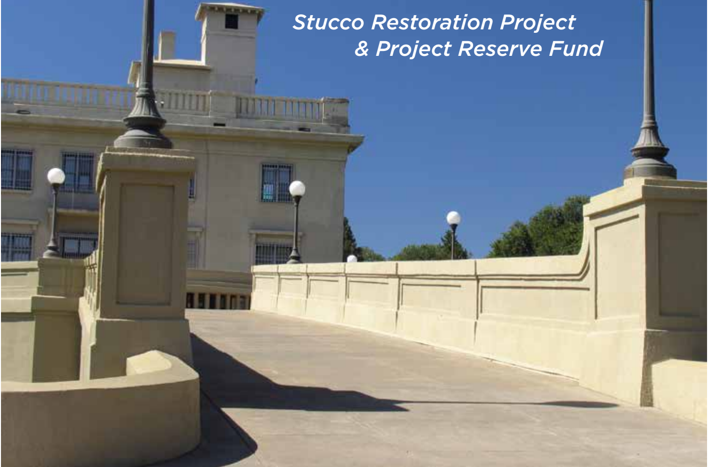
The East (Entrance) Ramp at Maryhill Museum of Art. Photo by Scott Thompson.
